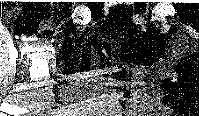
Step 3 The specially designed carriage is rolled into position.
